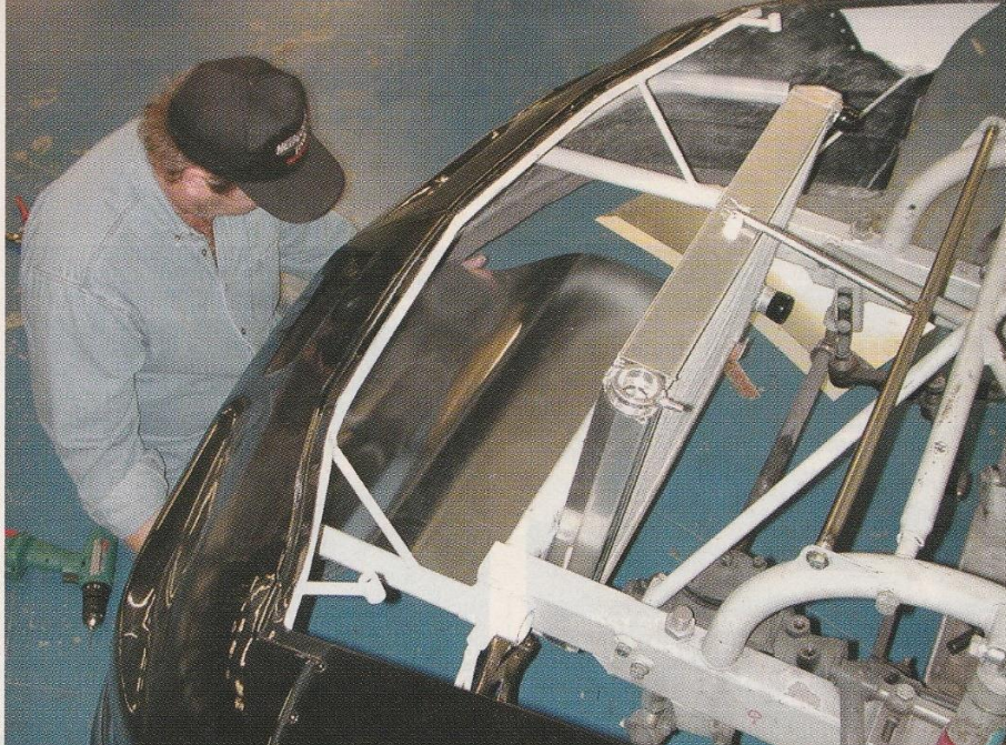
Davis test-fits the first section of the radiator box to make sure he is getting the curve he wants. This photo gives you a good idea of how the floor of the radiator box is shaped as well as how the top bracket holding the radiator in place is built.
